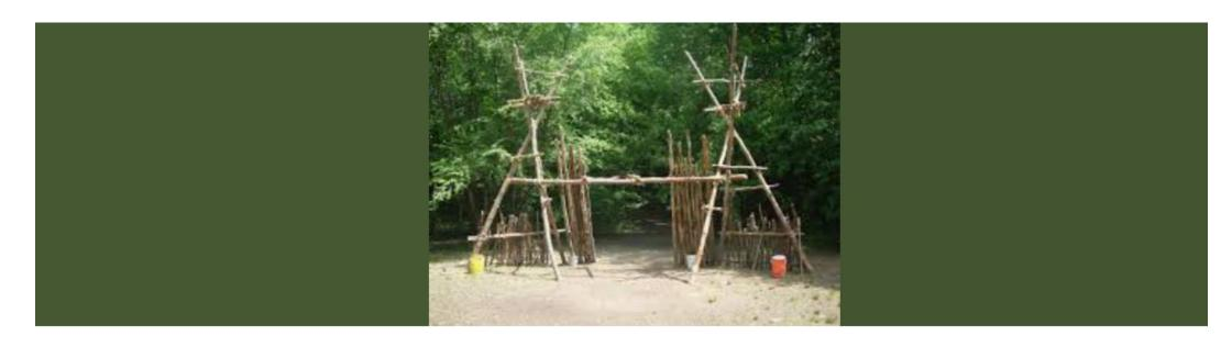
**Pioneering** is the art of using ropes and **wooden** spars **joined** by lashings and knots to create a structure. **Pioneering** can be used for constructing small items such as camp gadgets up to larger structures such as bridges and towers. These may be recreational, decorative, or functional.
